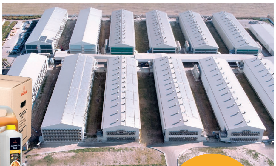
Laying farm complex in Stavyshe, Kyiv region, Ukraine
